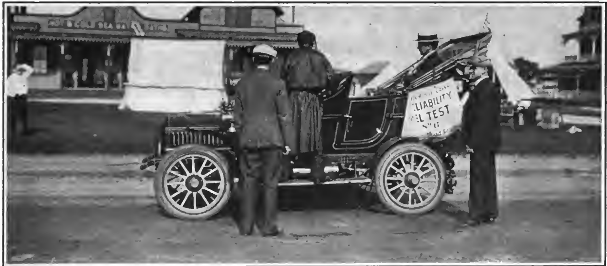
WAYNE TOURING CAR, ONLY "WATER-COOLED" IN CONTEST.—THIS MACHINE COVERED 1,902 MILES IN 145 HOURS, 2 MINUTES.
